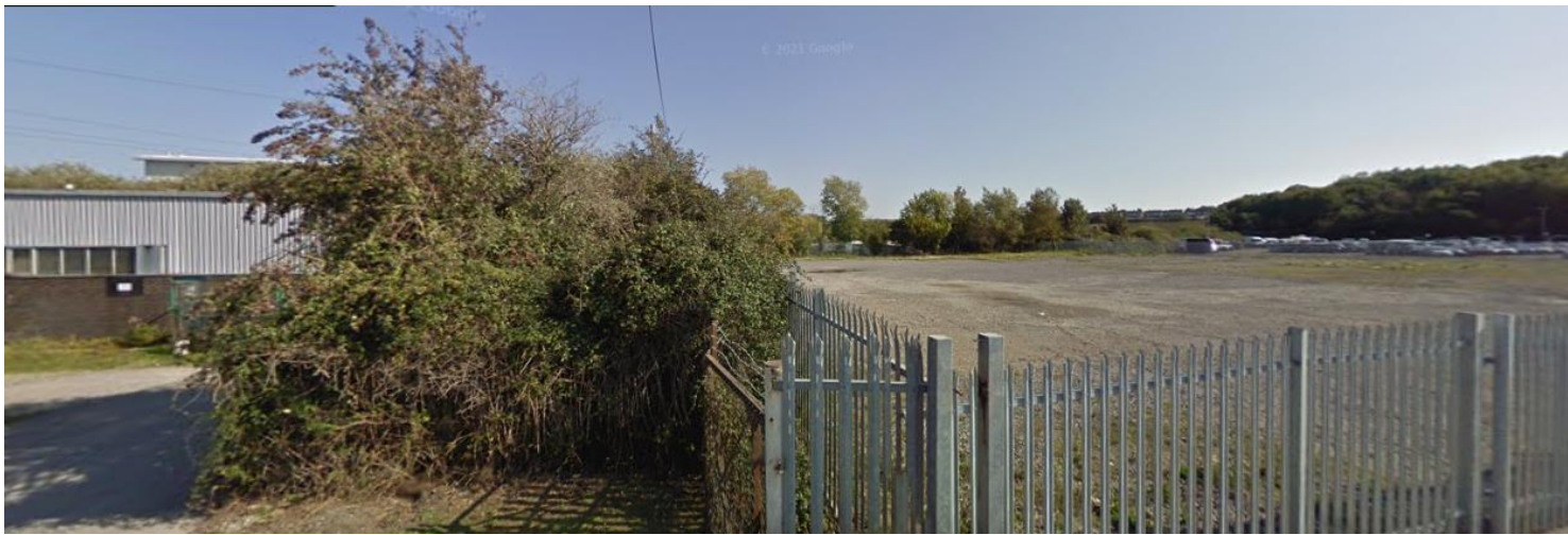
Looking east across the site from the West Wilts Trading estate
