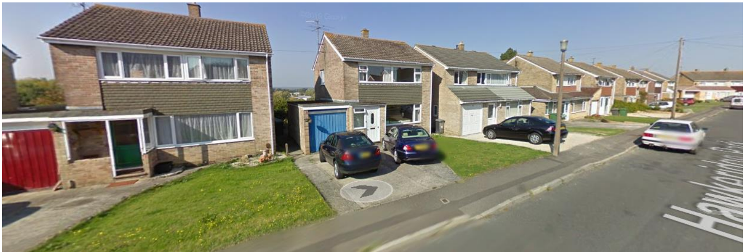
Hawkeridge park properties with the site beyond and west wilts trading estate in the distance
